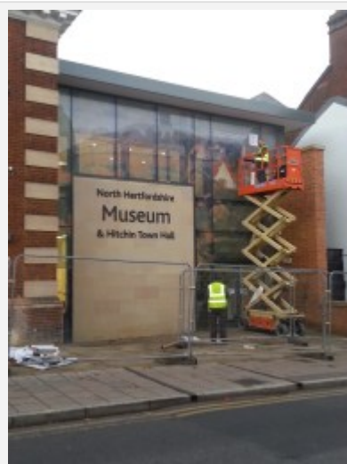
Using a scissor lift to attach the vinyl image
